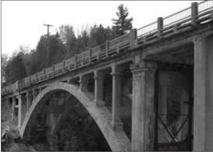
Historic Lime Kiln Bridge
