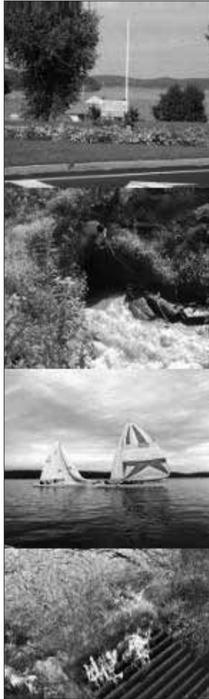
East Lakeshore Drive Stormwater Repair
