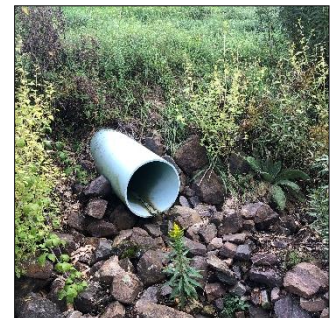
Drainage outfall in good condition
