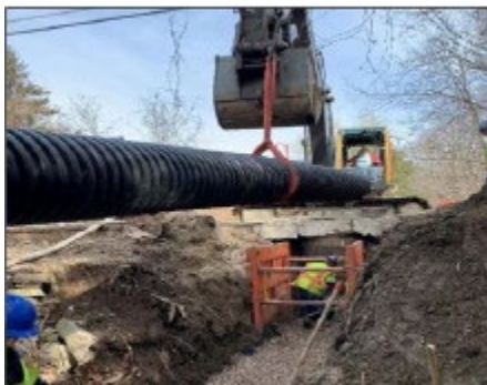
Recent Outfall Replacement Project on Williams Rd
