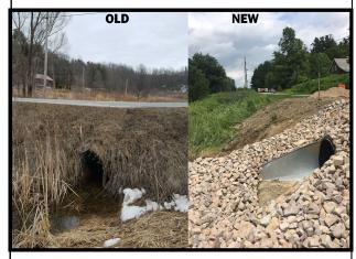
Above: A look at the recently completed culvert replacement project on East Road. The existing 36" metal culvert was removed and a 48" HDPE plastic culvert took its place, with the surrounding area stabilized to prevent erosion. The HDPE plastic has proven to be more resilient to the freeze-thaw cycle that happens each year, and the larger size allows more water to pass safely under the roadway, increasing our resiliency in the face of more frequent and extreme storm events.
