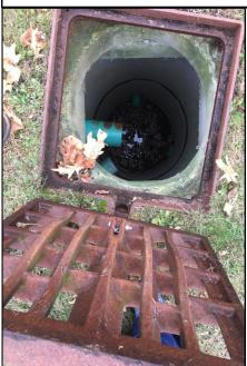
A look into a Town catch basin along Granite Creek Road. These systems collect rainwater that runs off driveways, roads, and building roofs during storms, and transports the stormwater directly to nearby rivers. streams, or Lake Champlain.
