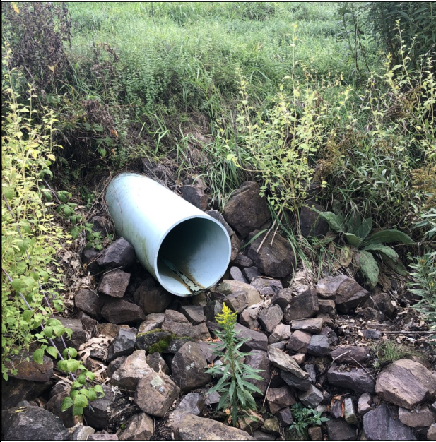
Above: Drainage outfall in good condition.
