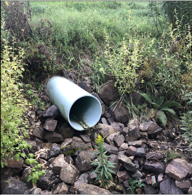
Above: Drainage outfall in good condition.
